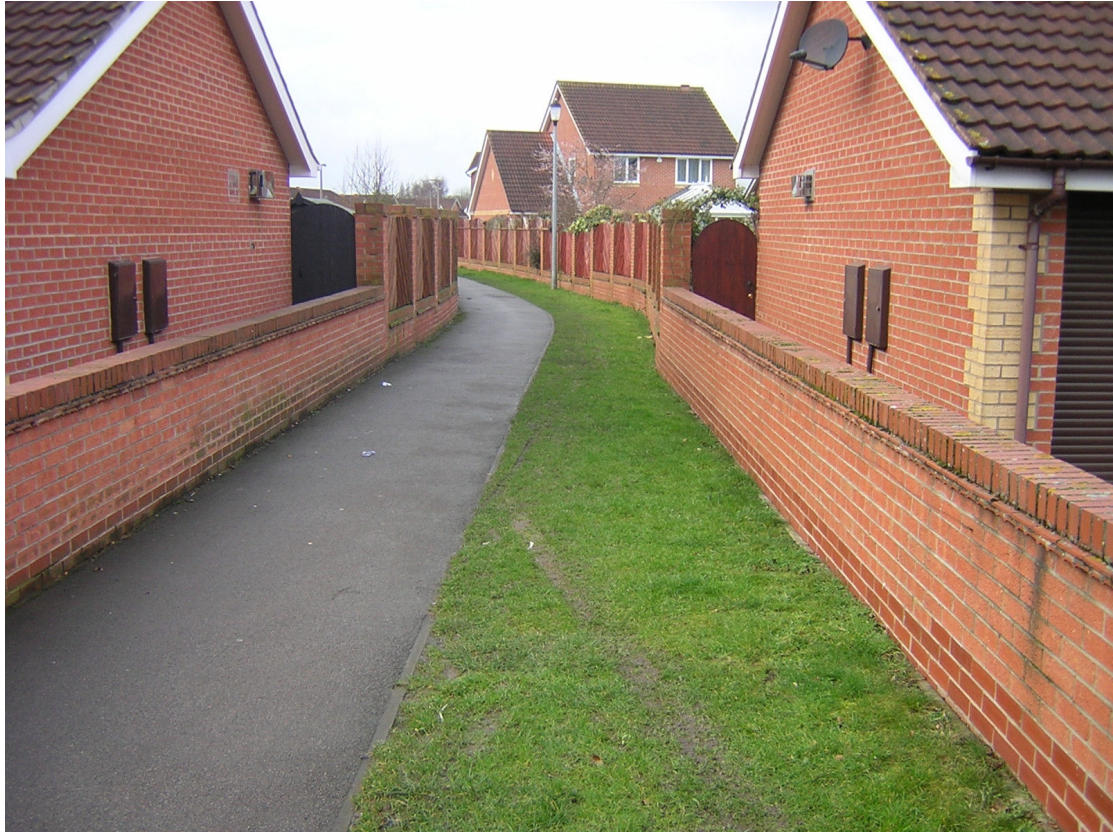
View from New Lane towards Stratford Way
