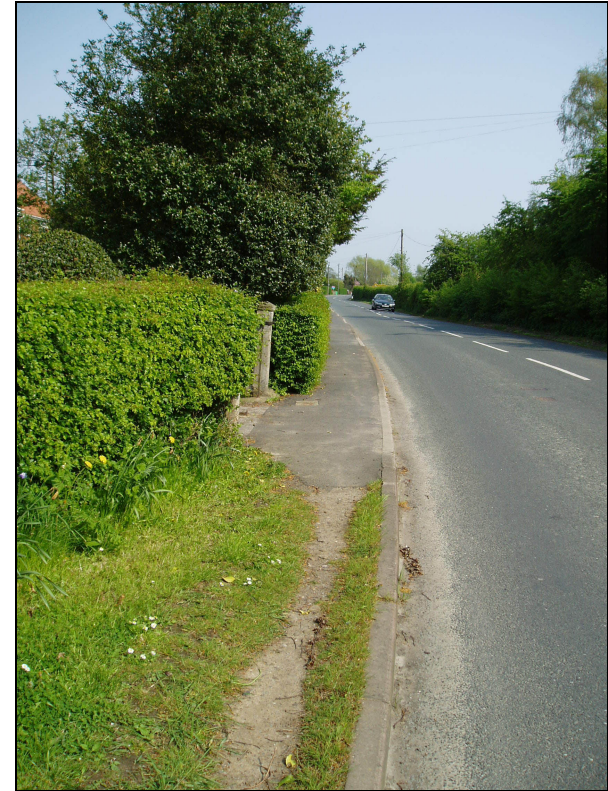
Figure 4 : Start of footway outside No. 107 Temple Lane
