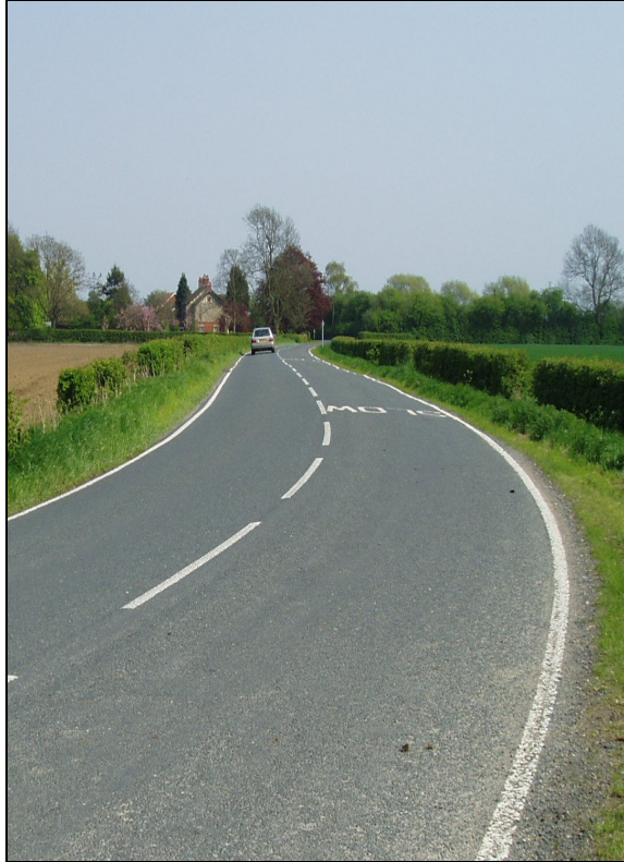
Figure 3 : Photograph showing the section of Temple Lane with no footway
